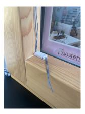
The last mounting shoe is on tension pull it and slide it over the remaining metal bracket.
